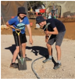
Nathan and James of C321 are digging a trench to bury their water supply hose under a road.
