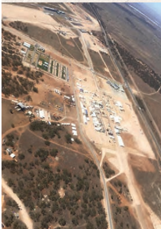
An aerial shot of the site. Photo: SCOUTS SA
